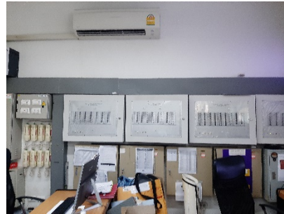
Graphic Annunciator Fire Alarm System
