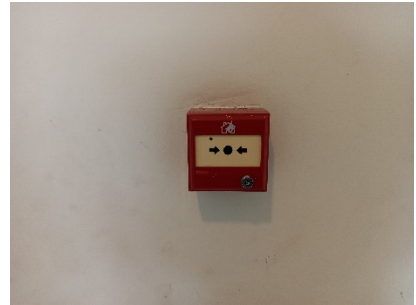
fire alarm manual station
